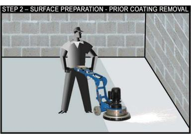
All previously coated surfaces must be ground to bare concrete by either shot-blasting or with a mechanical concrete grinder prior to application. It is imperative that all previous coating be completely removed and that the COOL-TEX® System be applied to bare concrete.
