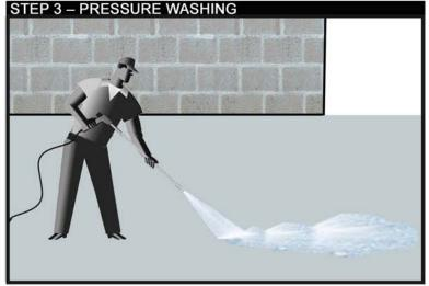
After acid etch and/ or previous coating removal, bare concrete surface should be power washed thoroughly with water pressure of at least 2000 PSI and allowed to dry.
